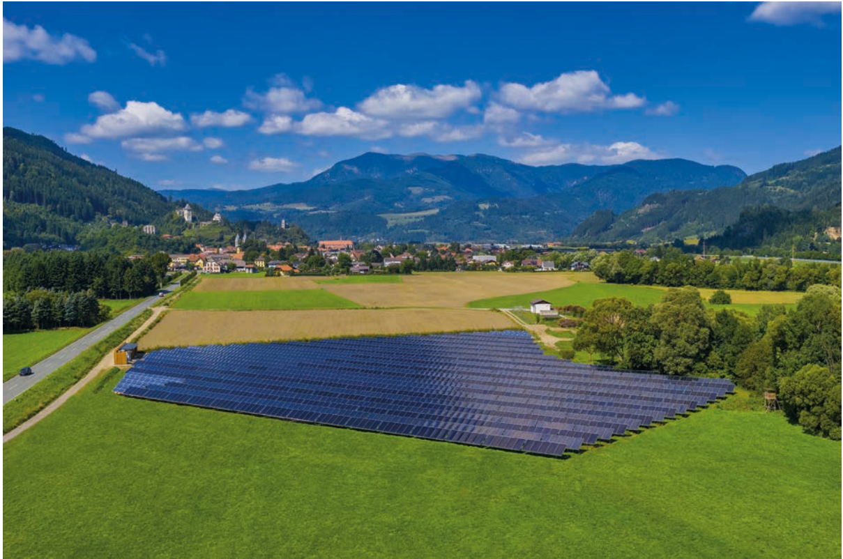
The Austrian solar district heating system in Friesach, with a capacity of 4.1 \text{ MW}_{\text{th}} , corresponding to 5,950 \text{ m}^2 flat plate collectors, was installed in 2021 Photo: Greenonetec Solar Industry GmbH, Austria
