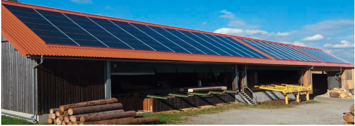
Solar wood chip drying with air collectors, Austria Photo: Austria Solar / CONA
