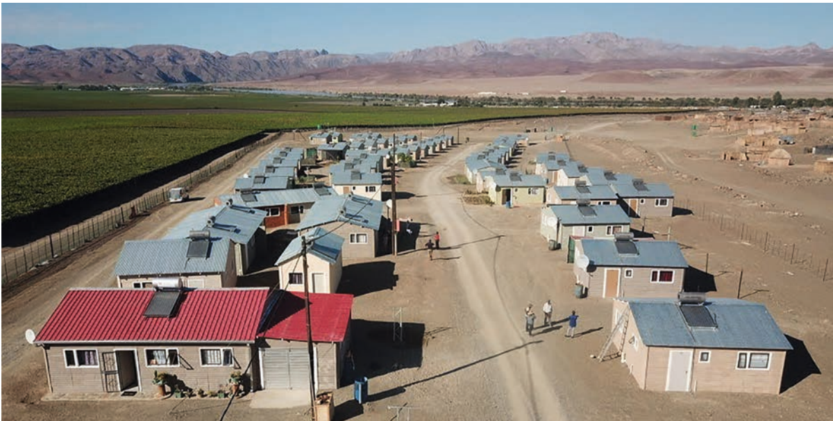
Aussenkehr, low-cost social housing project, Namibia
