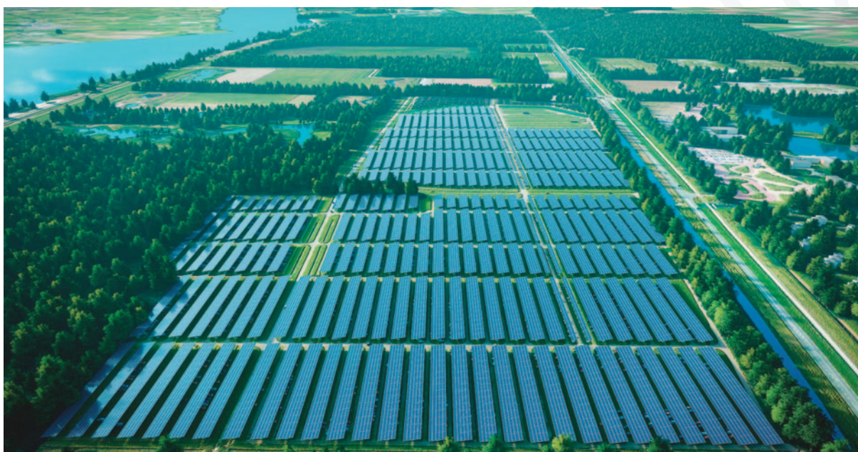
35 MW solar Carport, Dronten, Netherlands.
