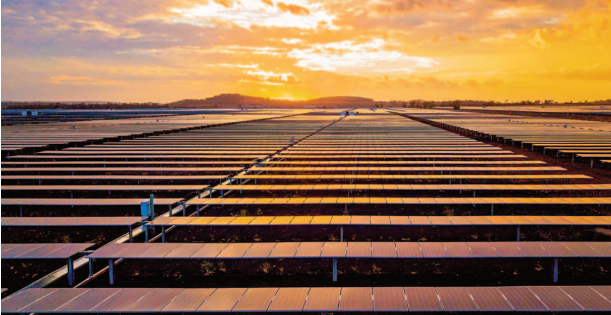
100 MW, Yarranlea Solar Farm, Queensland, Australia.
