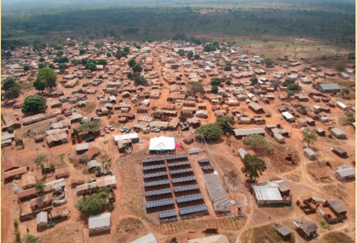
Budo Aare solar mini grid in Nigeria powered by a 100 kW PV-diesel hybrid system
