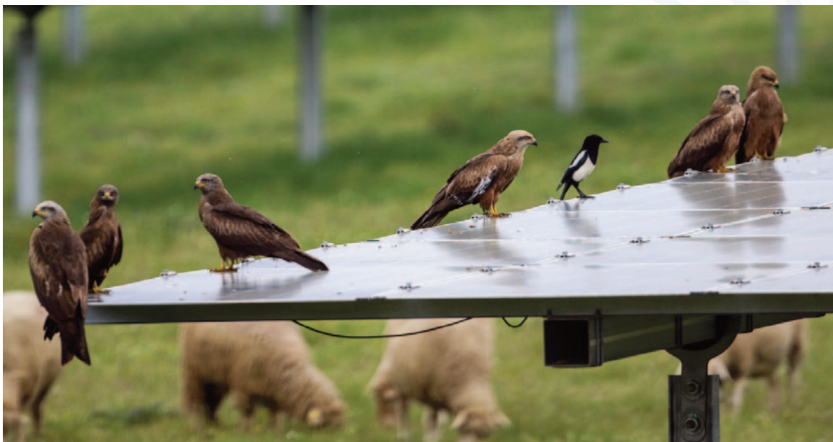
50 MW, Solanilla, Trujillo, Spain.
