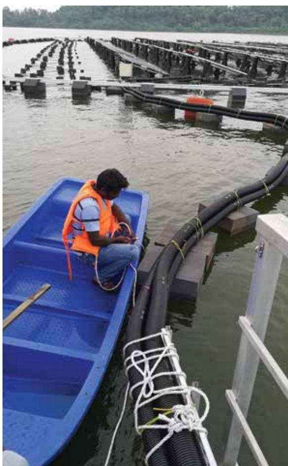
FIGURE 9.17 Maintenance on cables returning to shore
