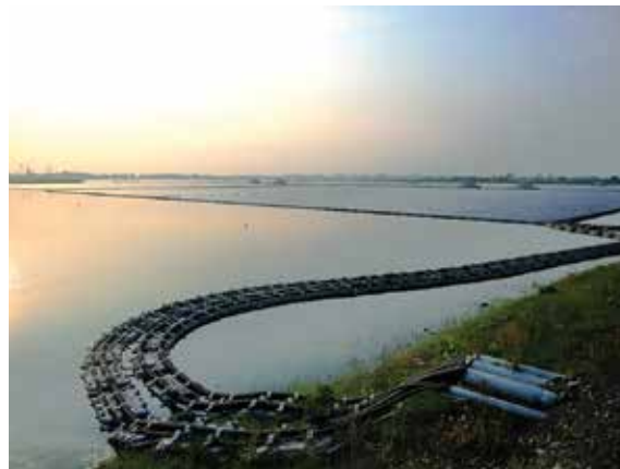
FIGURE 4.12 Cables routed to land from floating islands in MWp-scale FPV plants in Hyogo Prefecture, Japan (left), and in Anhui Province, China (right)
