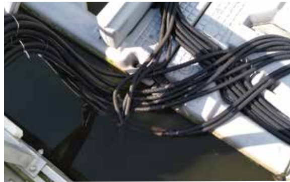
FIGURE 9.16 Biofouling on submerged connectors and cables
