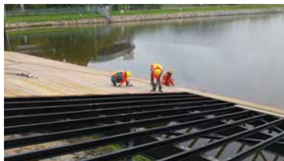
FIGURE 7.2 Construction of a launch ramp
