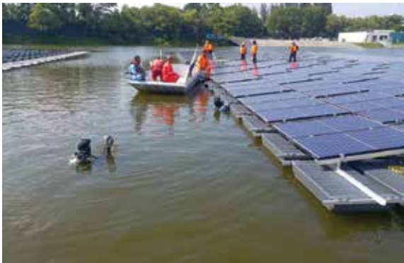
FIGURE 7.10 Professional divers tie knots, install marker buoys, and anchor an FPV system (left); special barge used for anchoring and mooring system (right)
