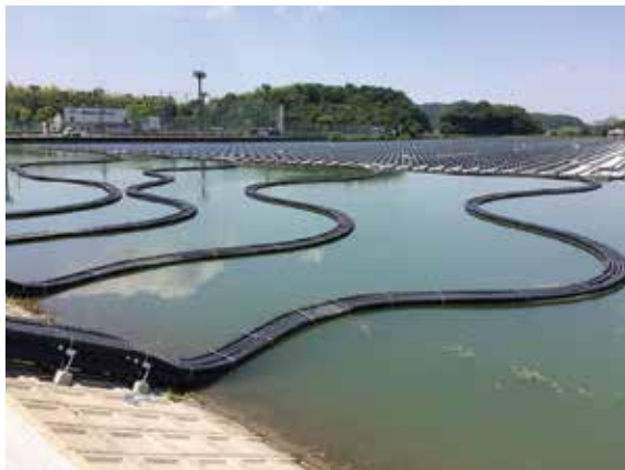
FIGURE 4.12 Cables routed to land from floating islands in MWp-scale FPV plants in Hyogo Prefecture, Japan (left), and in Anhui Province, China (right)
