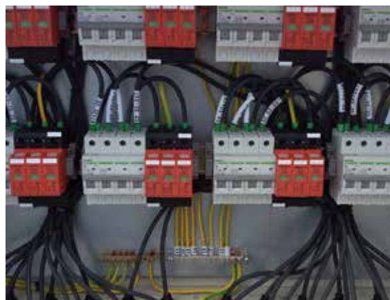
FIGURE 8.2 DC cabinet with surge protection devices (red-orange)
