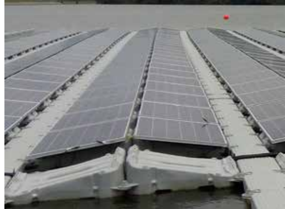
FIGURE 9.13 Floats on left side: modular and detachable from support structure; floats on right side: inter-linked, aligned, and secured to neighboring floats with a nut and bolt
