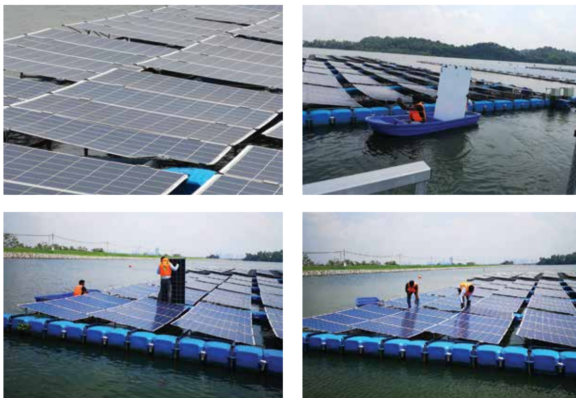
FIGURE 9.8 Replacement of a damaged solar module
