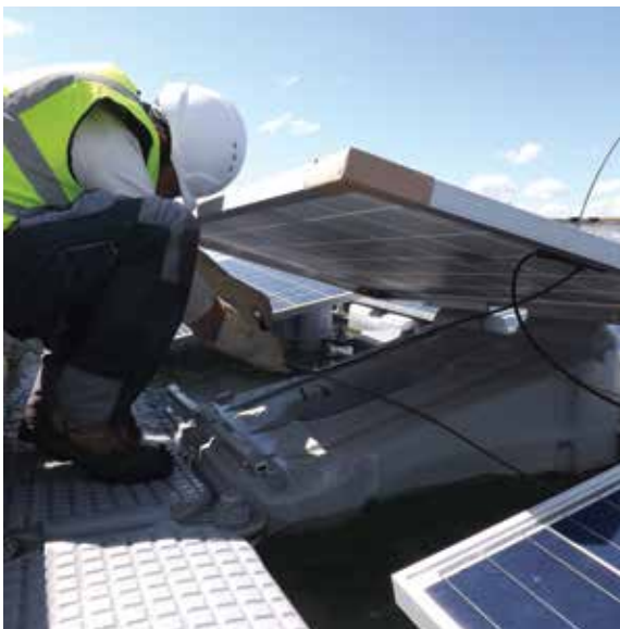
FIGURE 9.14 Corrective maintenance carried out on the float
