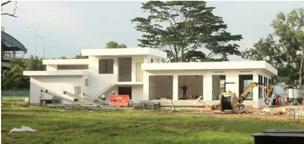
FIGURE 7.13 A substation under construction
