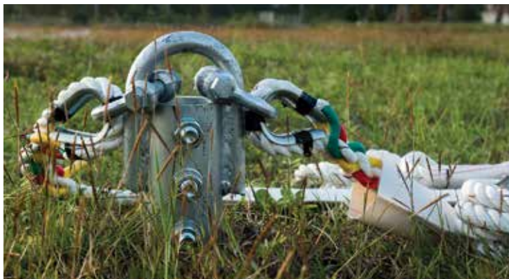
FIGURE 7.11 Land-based anchoring on the banks
