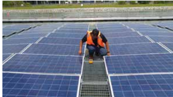
FIGURE 8.5 Solar professional performing continuity tests
