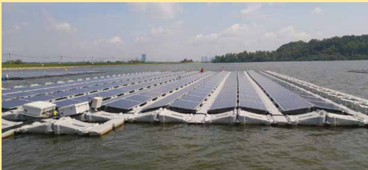
FIGURE 4.3 Dual-pitch configuration reduces wind load on FPV modules/systems
