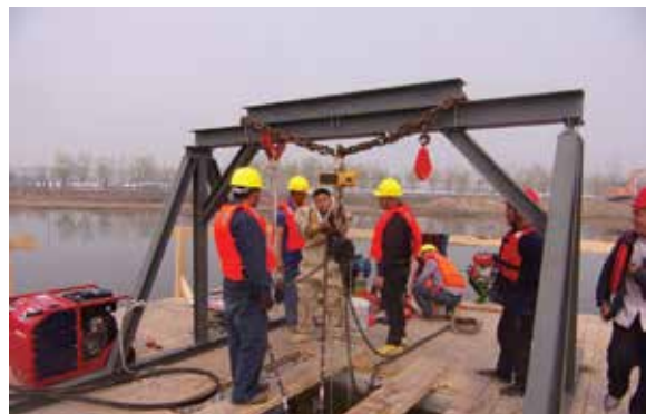
FIGURE 7.10 Professional divers tie knots, install marker buoys, and anchor an FPV system (left); special barge used for anchoring and mooring system (right)
