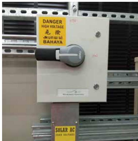
FIGURE 8.10 AC isolator
