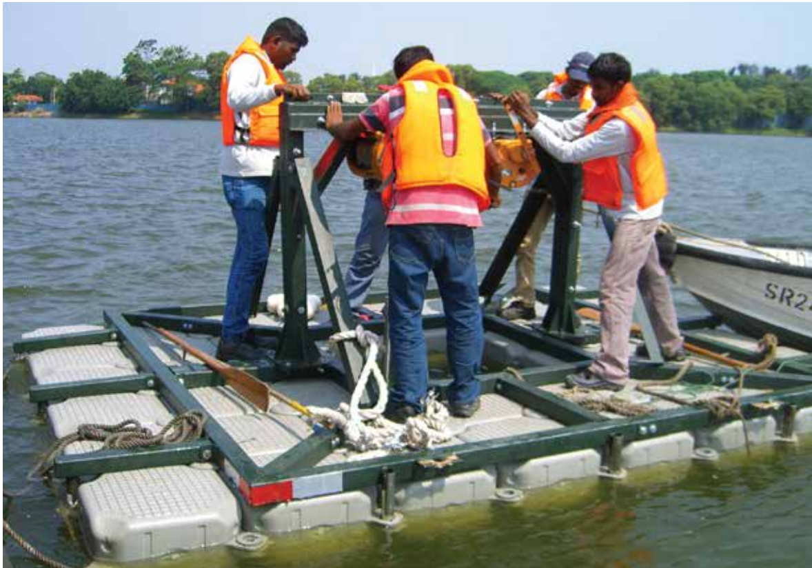
FIGURE 2.7 Concrete sinker test, Singapore Tengah Reservoir testbed
