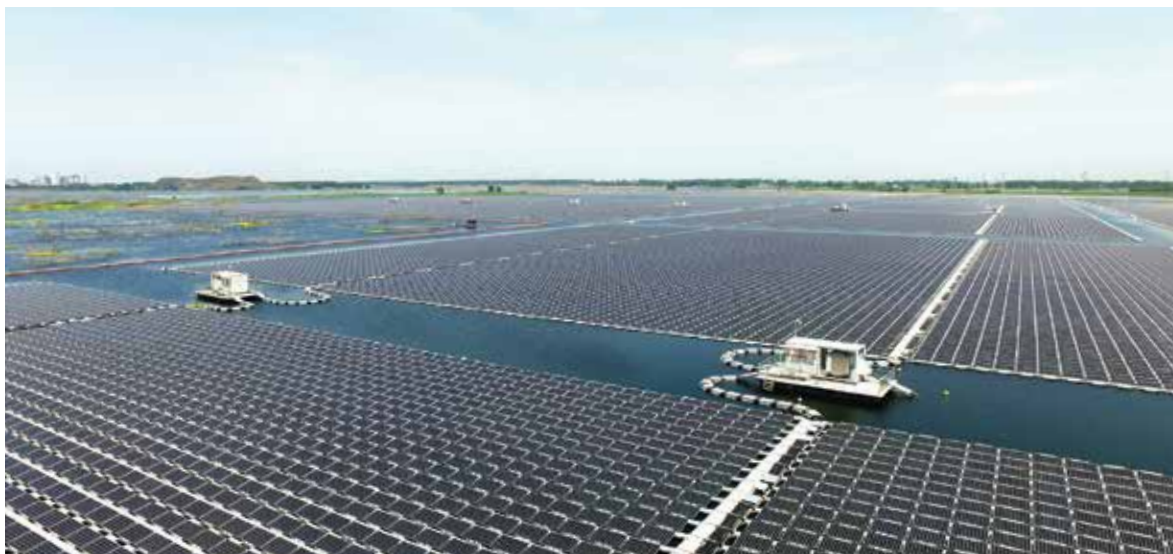
FIGURE 4.1 Central-inverter configuration for FPV systems, China
