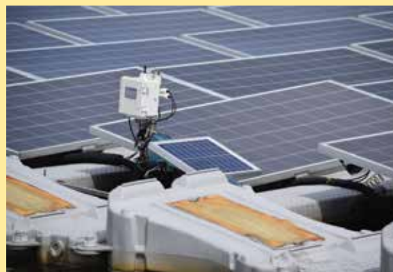
FIGURE 9.12 Sealing tape to cover open areas in floats
