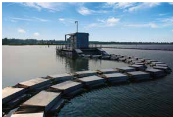
FIGURE 7.8 Main cable trunk routed to shore using floats (left), and floating by itself (right)
