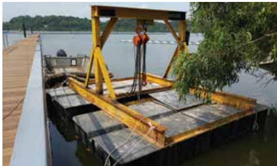
FIGURE 7.9 Barge used to lower concrete sinkers
