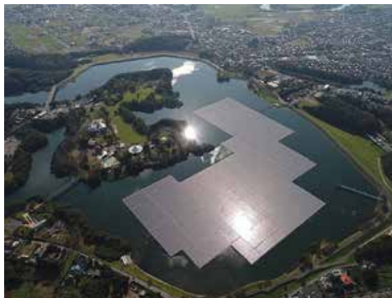
FIGURE 6.1 Glare on Yamakura dam in Japan
