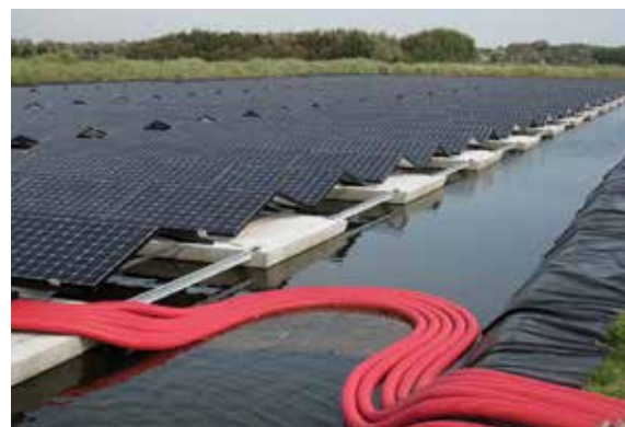
FIGURE 7.8 Main cable trunk routed to shore using floats (left), and floating by itself (right)
