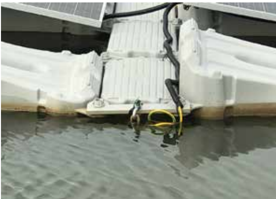
FIGURE 8.4 Grounding to reservoir bed
