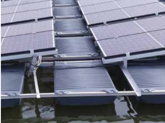
FIGURE 9.13 Floats on left side: modular and detachable from support structure; floats on right side: inter-linked, aligned, and secured to neighboring floats with a nut and bolt
