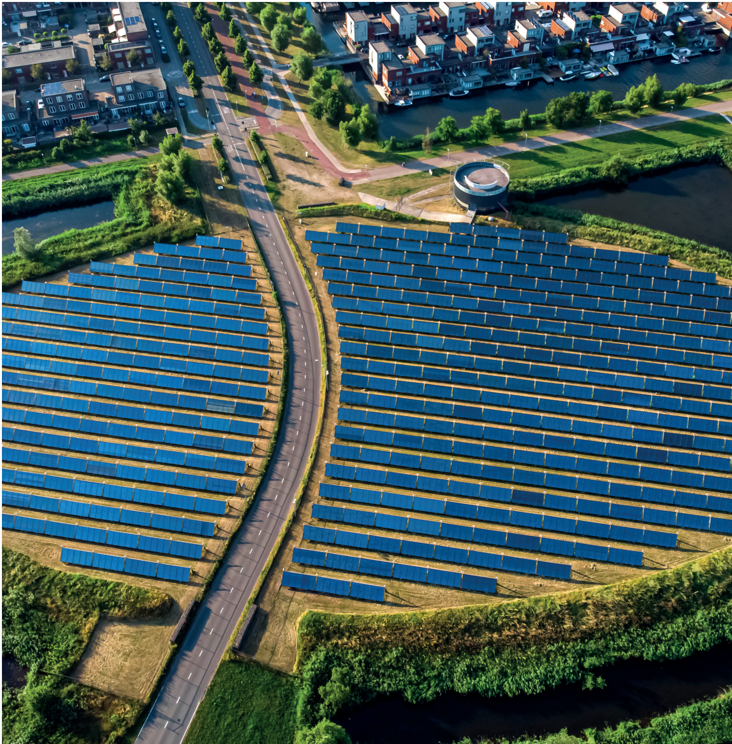
Solar Panel Farm with unique design in a form of an island (Zoneiland). Energy is used to power city heating (stadswarmte) in a modern sustainable district Noorderplassen in Almere, The Netherlands.
