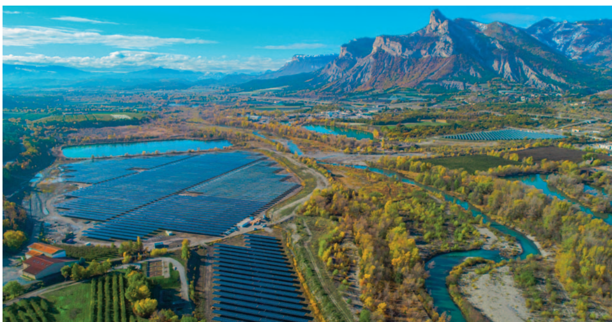
15 MW, Curbans, France.
