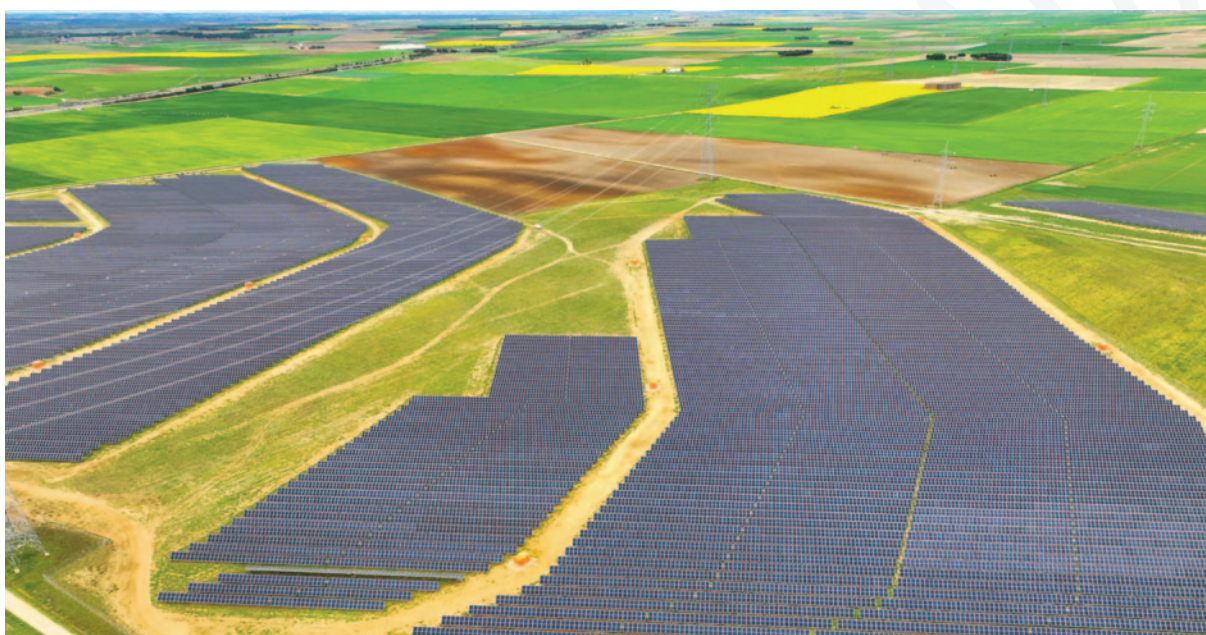
41.7 MW, Tordesillas, Spain.
