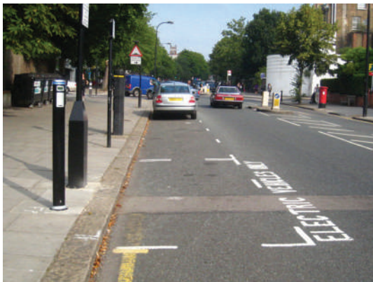
Figure 7.1 Charging point on the roadside (Source: Rod Allday, http://www.geograph.org.uk )
