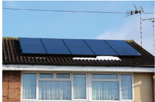
Figure 7.26 A 4kW array of PV panels (ten front and six more at the back)
