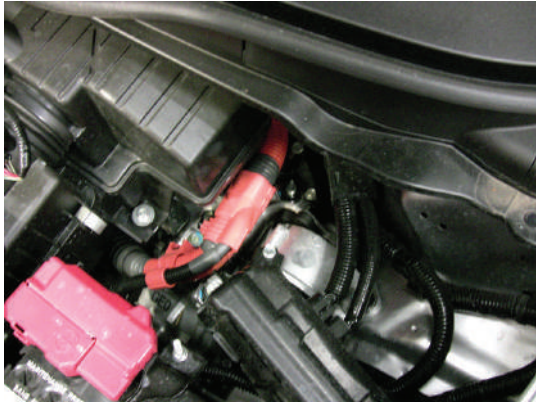
Figure 2.6 High-voltage cables are always orange
