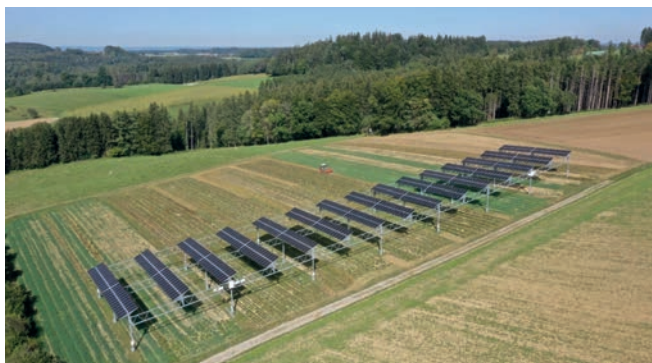
Fig. 50: Agrivoltaic system in Heggelbach with a capacity of 194 kW p covering approximately a third of a hectare.
