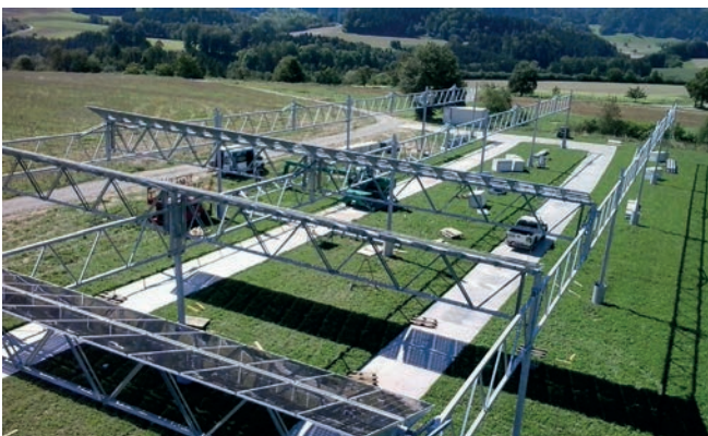
Fig. 53: Construction roads to avoid soil compaction. © BayWa r.e.
