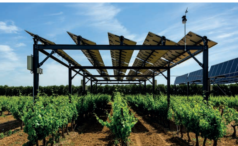
Fig. 26: Agrivoltaic system with solar tracking PV modules in France. © Sun'Agri
