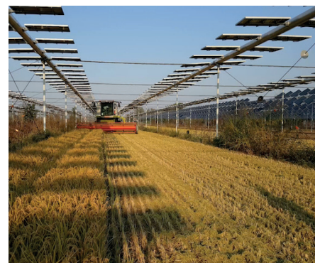
Fig. 43: Overhead systems with narrow PV modules in Italy. © REM Tec
