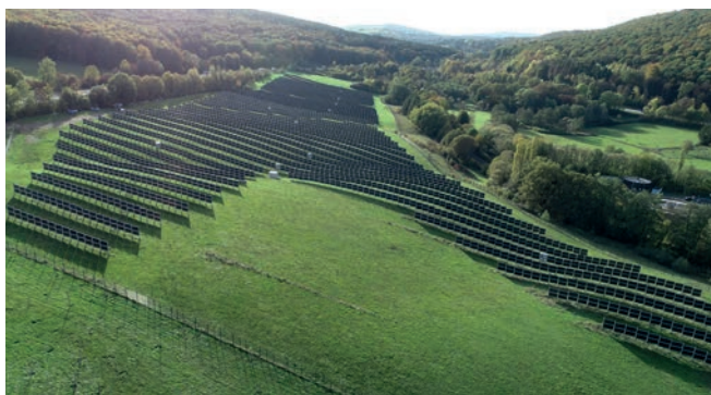
Fig. 51: Eppelborn-Dirmingen solar farm with 2 MW p with vertical solar fences by Next2Sun. © Next2Sun GmbH
